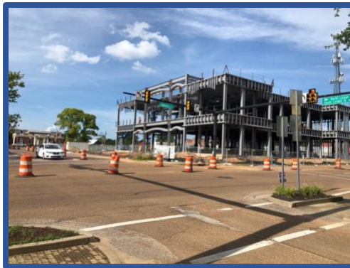
Definitely a building project!
